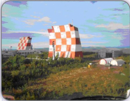
Soil samples were collected at the Kalakaket Creek radio relay station. The site is accessible only by helicopter.
