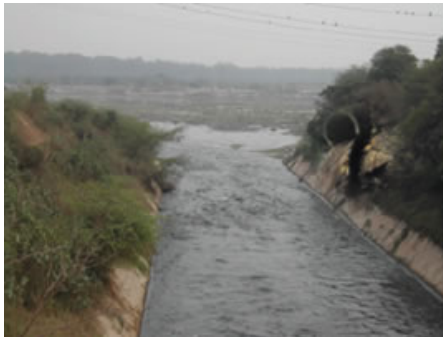
Delhi Interceptor Sewer Project Yamuna River, Delhi
